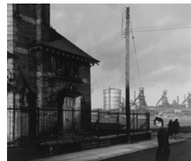
Graham Smith Clay Lane Furnaces. South Bank, Middlesbrough. 1981
